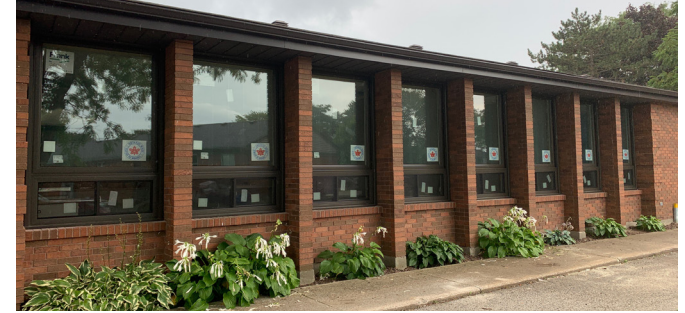
New windows installed by St. Clair Township at Sombra Library.
